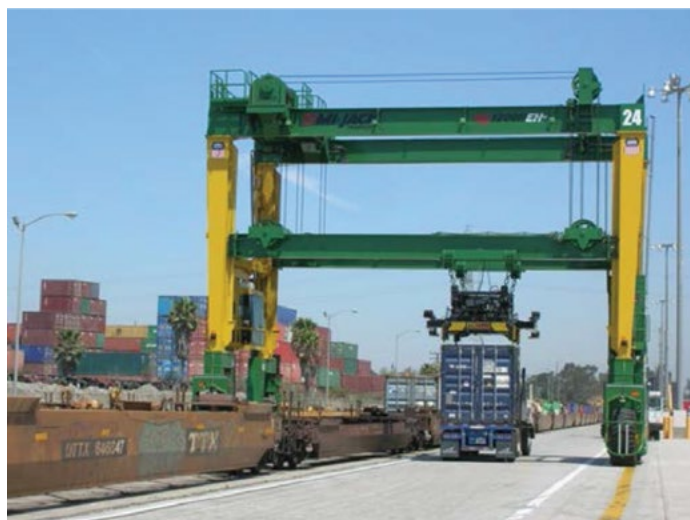
Figure 3: Mi-Jack Products has developed a freight yard management system that greatly improves the efficiency of goods transfers, reduces truck idling, eliminates emissions from cranes, and allows for more compact freight yards in established industrial areas.
