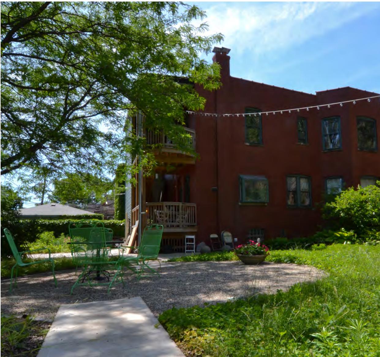
A RainReady apartment building
