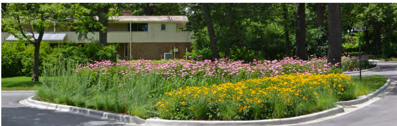
A RainReady street with bioswale to capture stormwater runoff
